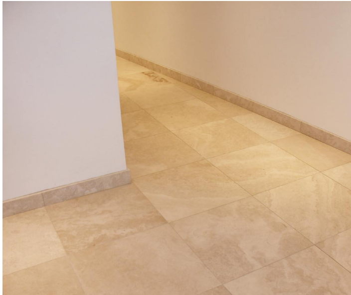
Custom cut skirting has been manufactured to match the tiling joints of the 60x60cm GOSS Artemis limestone tiles.
