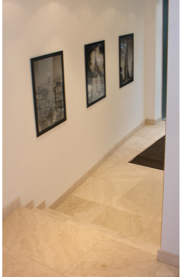
Custom cut skirting has been manufactured to match the tiling joints of the 60x60cm GOSS Artemis limestone tiles.
