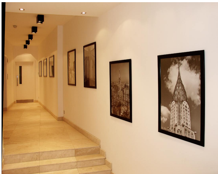
Custom cut skirting has been manufactured to match the tiling joints of the 60x60cm GOSS Artemis limestone tiles.
